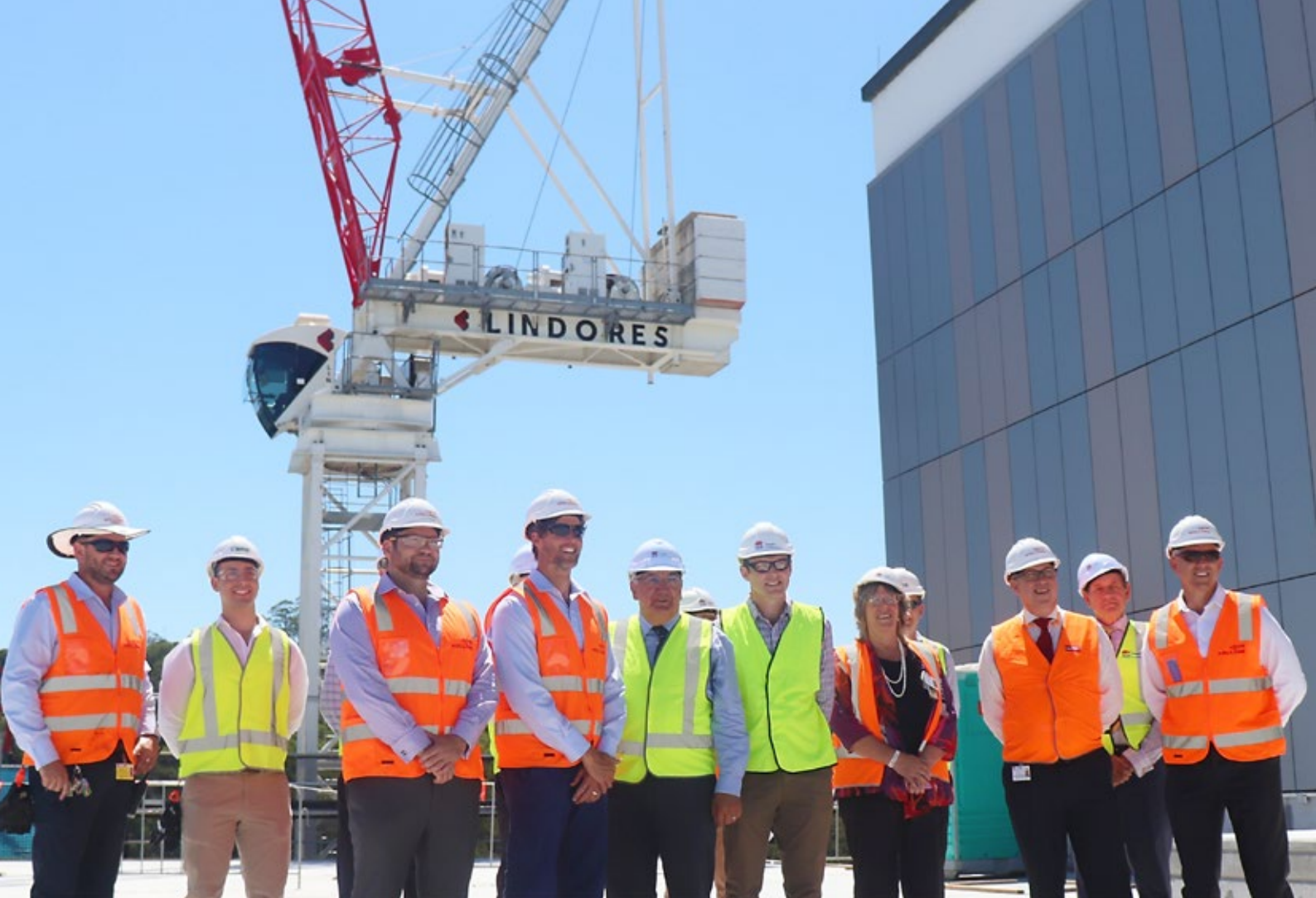
Redevelopment project staff with Member for Lismore, Thomas George (centre), and Northern NSW Local Health District management and Board members at the Lismore Base Hospital North Tower 'topping out' ceremony.
