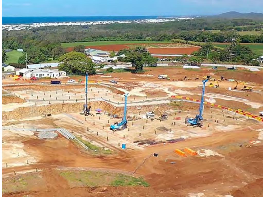
Tweed Valley Hospital construction site
